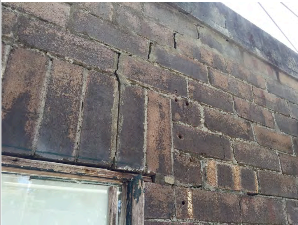
Large cracks above the window to the right side of the detached garage extending into the roof slab.
