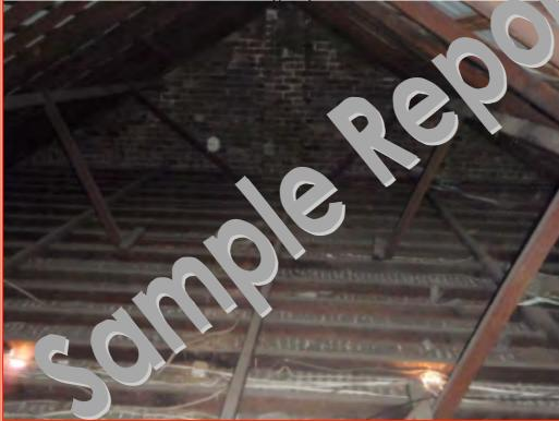
An excessive build-up of dust and debris was noted to the roof void area. This material is potentially a health hazard and should be removed.
