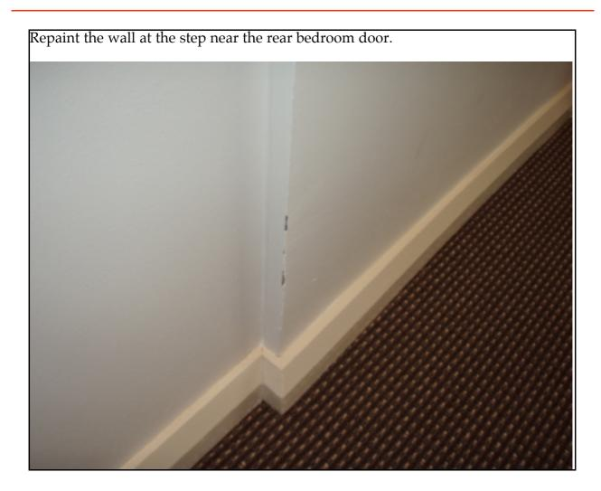
Repair the poorly finished, out of square wall lining and skirting board to the rear upper bedroom.
