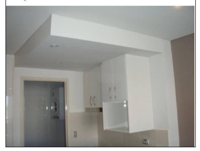
Seal the join between the kitchen wall cupboard and the wall lining above the microwave oven shelf.
