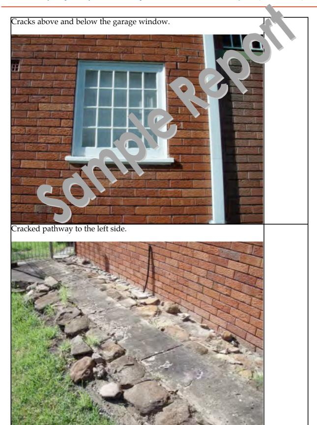
Cracks above and below the left side window to the room at the rear of the garage.
