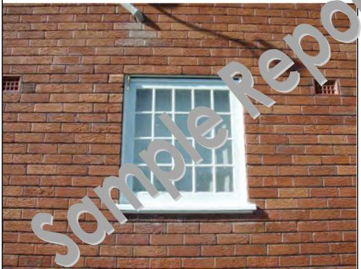
Cracks noted to the brickwork above and below the left side upper level window.
