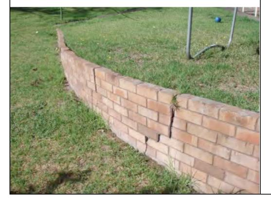
Several cracks noted to the brick retaining wall to the left side of the property.
